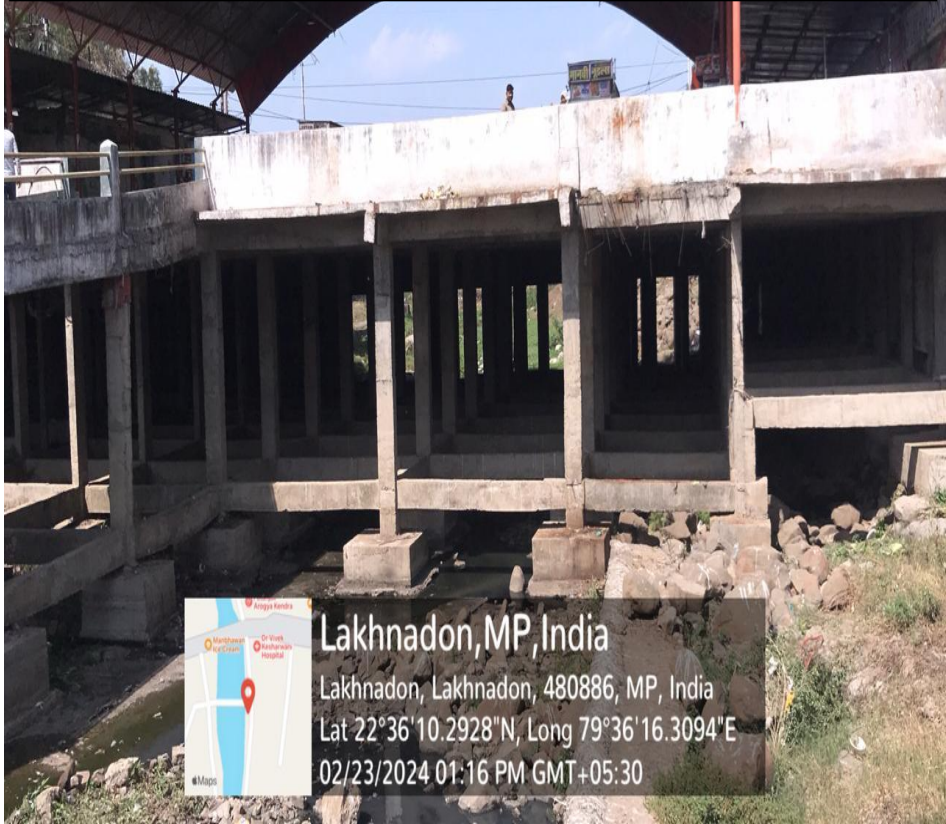
FOUNDATION OF CHAUPATI SHOWING NUMEROUS BEAMS & COLUMNS
